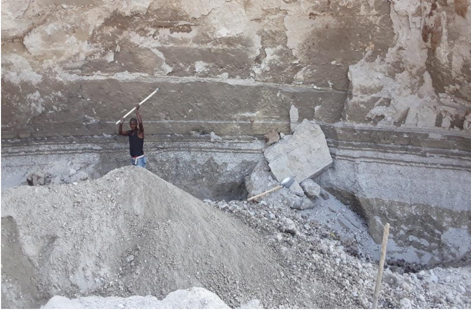
Figure 10: Photo of sands excavated from borrow pit at Ituha area.
